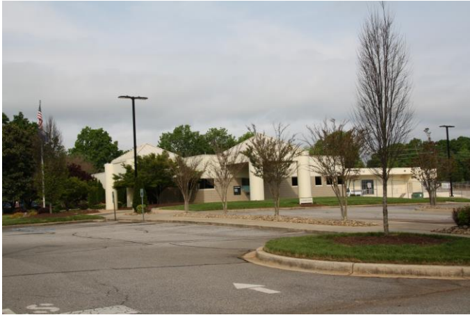
WEST – Utility company adjacent to west of site Facing west from parking lot near edge of site Site is to the right of building
