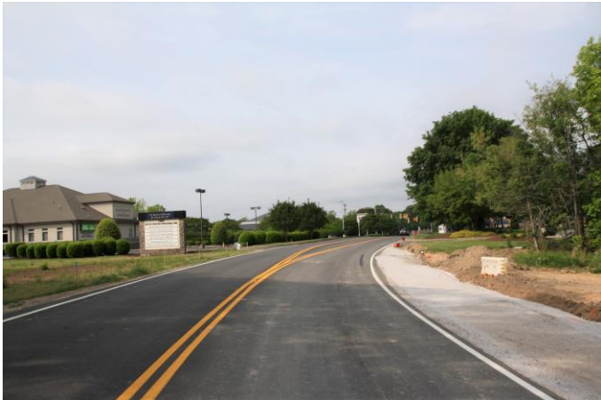
STREET – Facing southwest along E. Butler Road Site is undeveloped property to the right Medical offices can be seen in distance on the left
